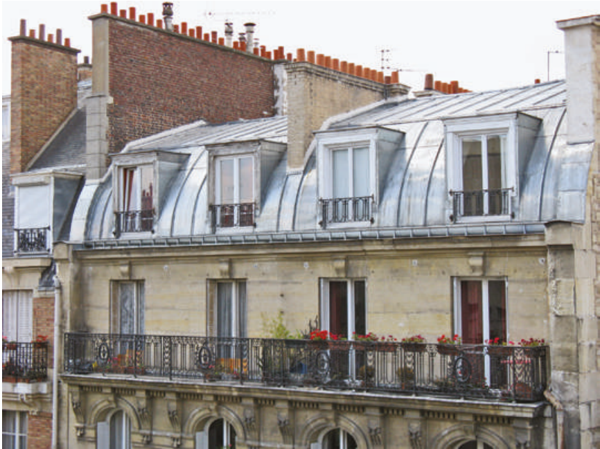
Figure 2.19 Rooftop chambres de bonne in Paris, 2008. Photograph by Rafael Garcia-Suarez via Wikimedia Commons.
