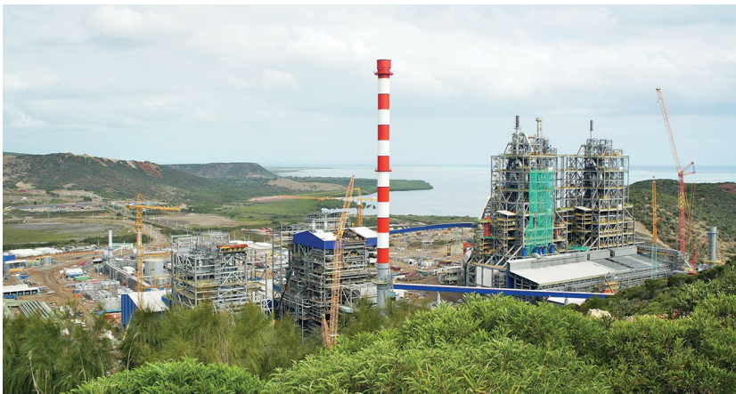
Figure 3.1 The Koniambo project construction site, September 2012.
