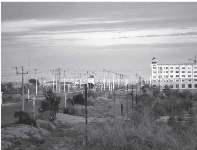
Fig. 10 Wind turbines and the town's electric power station (Ereen city, August 2010). Photo: G. Lacaze.
