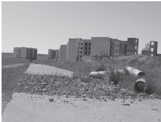
Fig. 5 Ruined buildings and roads (photo: S. Batchimeg, 2009)
