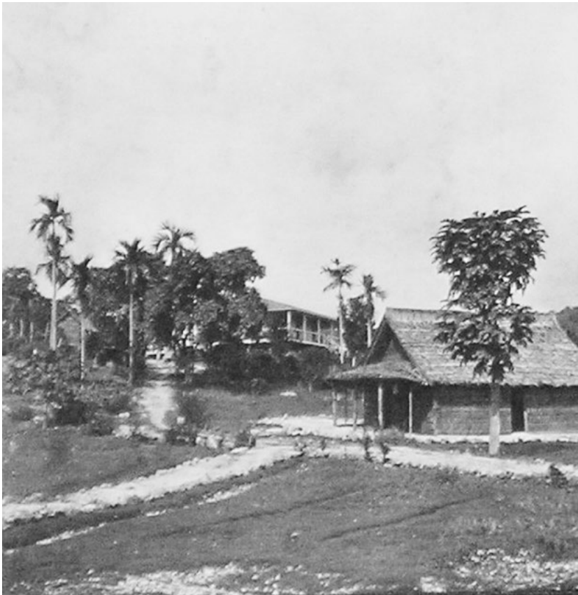
Figure 7.1: The residency, the Malaita resident magistrate's (later the district officer's) house, and the office built for Thomas Edge-Partington in 1910.
