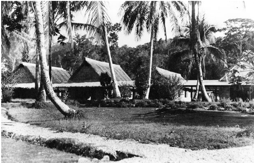
Figure 10.4: Hospital of the Epiphany at Fuaaabu, northwest Malaita in the 1930s.
