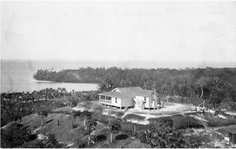
Figure 7.2: The police commander's house at `Aoke, built for Frederick M. Campbell in 1912.
