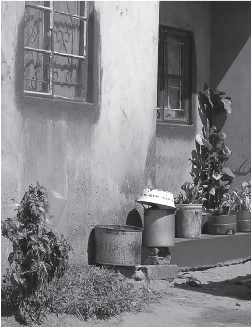
Fig. 1.3 Front entry of a house in George showing some of the details children identified with pride. The entryway and flowerpots were polished in a deep red. The windows were outlined with the same red polish. Photo by Rosha Forman.
