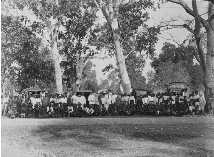
Figure 14. Official opening of (unsealed) Kupang-Atambua road, 1923 (KITLV image nr. 11147).
