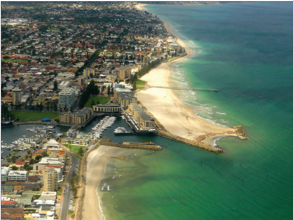
Figure 2.12 The Patawalonga Estuary, marina and breakwaters, showing residential development on reclaimed land and sand build on the south (upper) side with downdrift narrow beach on the north (lower) side.
