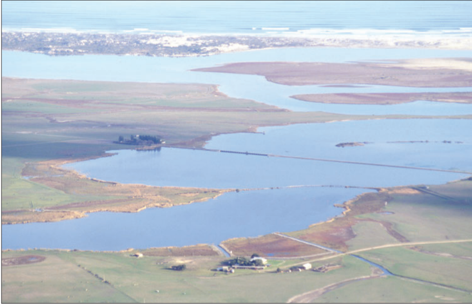
Figure 4.19 View across the Mundoo Channel, Mundoo Barrage and Bird Island to Younghusband Peninsula and the ocean. Only a small portion of Mundoo Barrage has operable gates to allow flows through, the remainder being a causeway. An early wooden curved barrage structure, built in 1915, is also visible.
