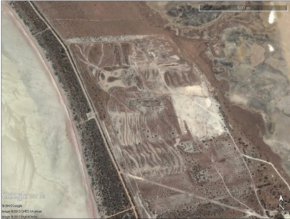
Figure 6.9 The coast north of Parham, illustrating a wide intertidal flat and a vegetated beach ridge sequence, behind which is the 'Windsor Farm' shell grit mining and rehabilitation, indicating an artificial pattern of ridge rehabilitation related to the mining process.
