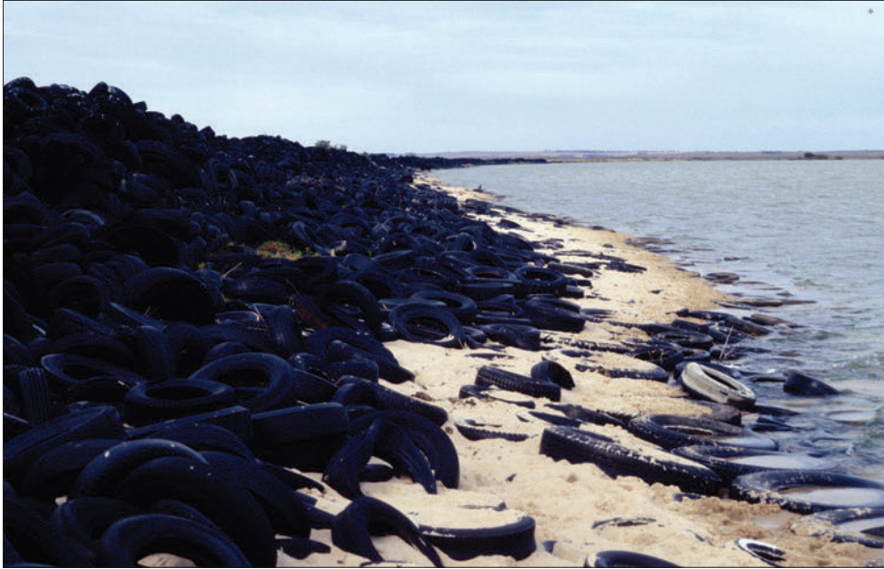
Figure 4.24 A tyre wall on part of the northwestern shoreline of Lake Alexandrina installed to inhibit shoreline erosion.
