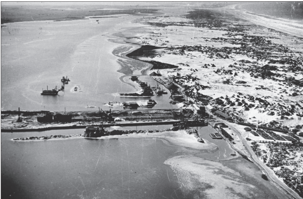
Figure 4.10 Sir Richard Peninsula during construction of the Goolwa Barrage in the 1930s. Large areas of drifting sand related to the effects of sheep, cattle and rabbits were infilling the Goolwa Channel. Compare with Figure 4.7.
