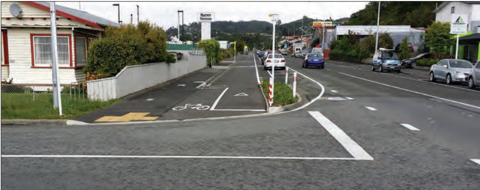
Figure 12.8: A separated cycleway with some ambiguity over side-road priority, in Nelson, New Zealand. (Source: Author.)
