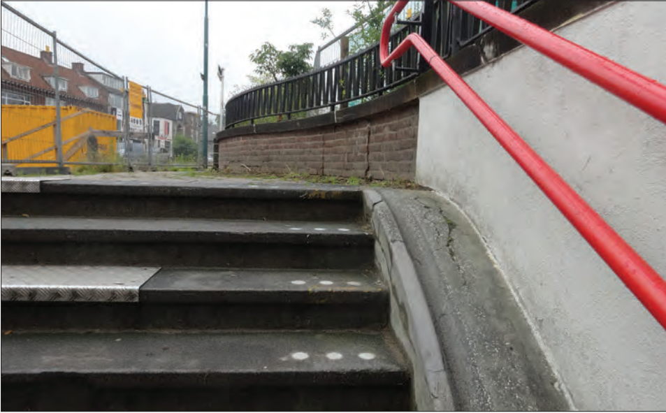
Figure 16.10: Integrated bicycle access ramp. (Source: author's own work.)
