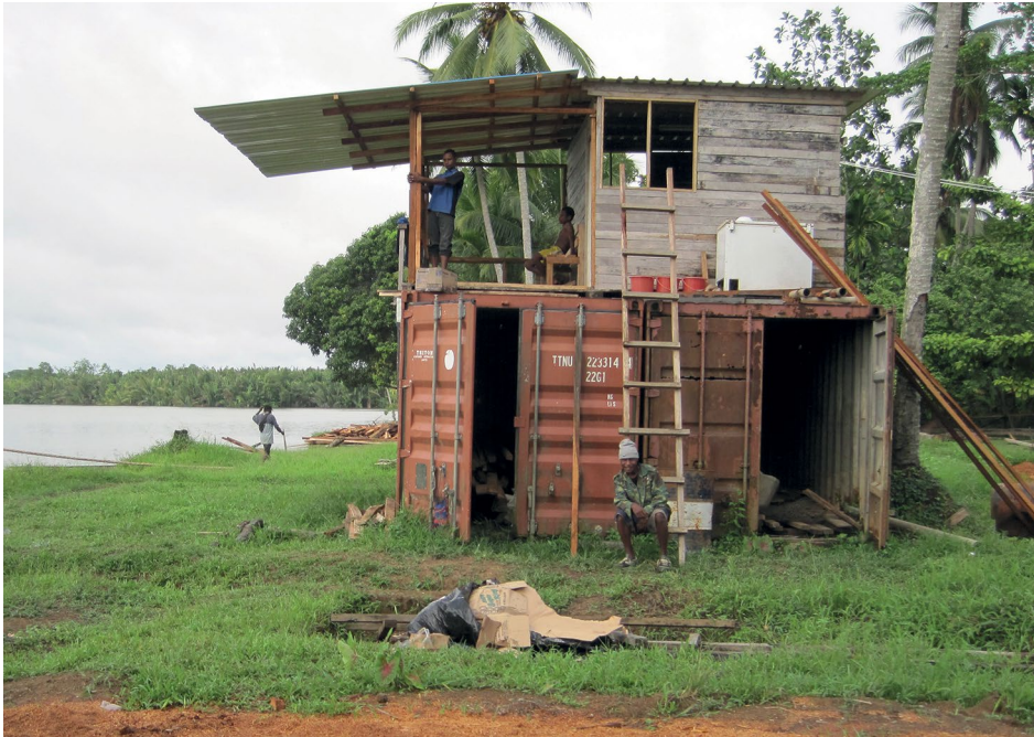
Figure 6.3 Containers on the bank of the Pie River used to form a security tower outside a Chinese-run trade store in Baimuru.
