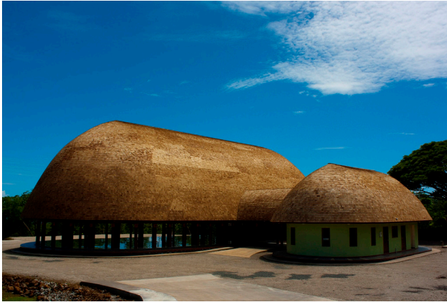
Figure 27. A modern version of a traditional Samoan fale recently constructed at the National University of Samoa
