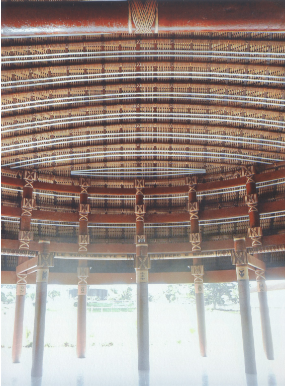
Figure 28. The interior lashings and construction details of the fale at the National University of Samoa
