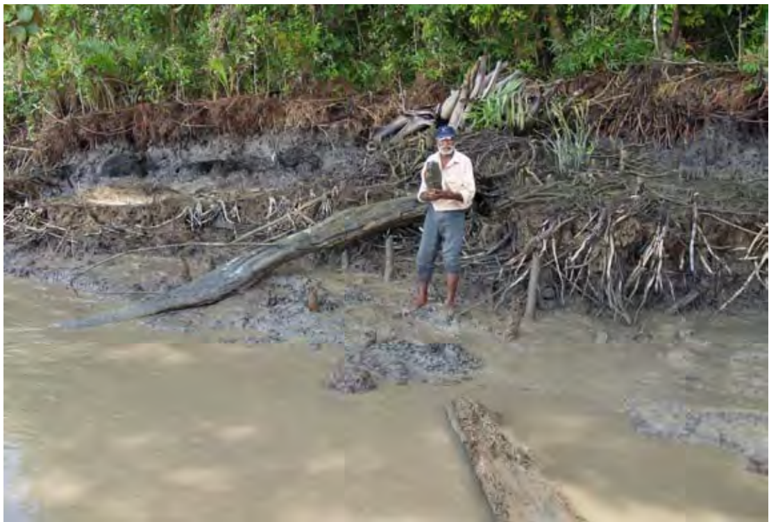
Figure 4. In situ longhouse posts at Otoia, exposed by tidal erosion. Note collapsed bank behind Hansen Iburi and the presence of posts behind the collapse.
