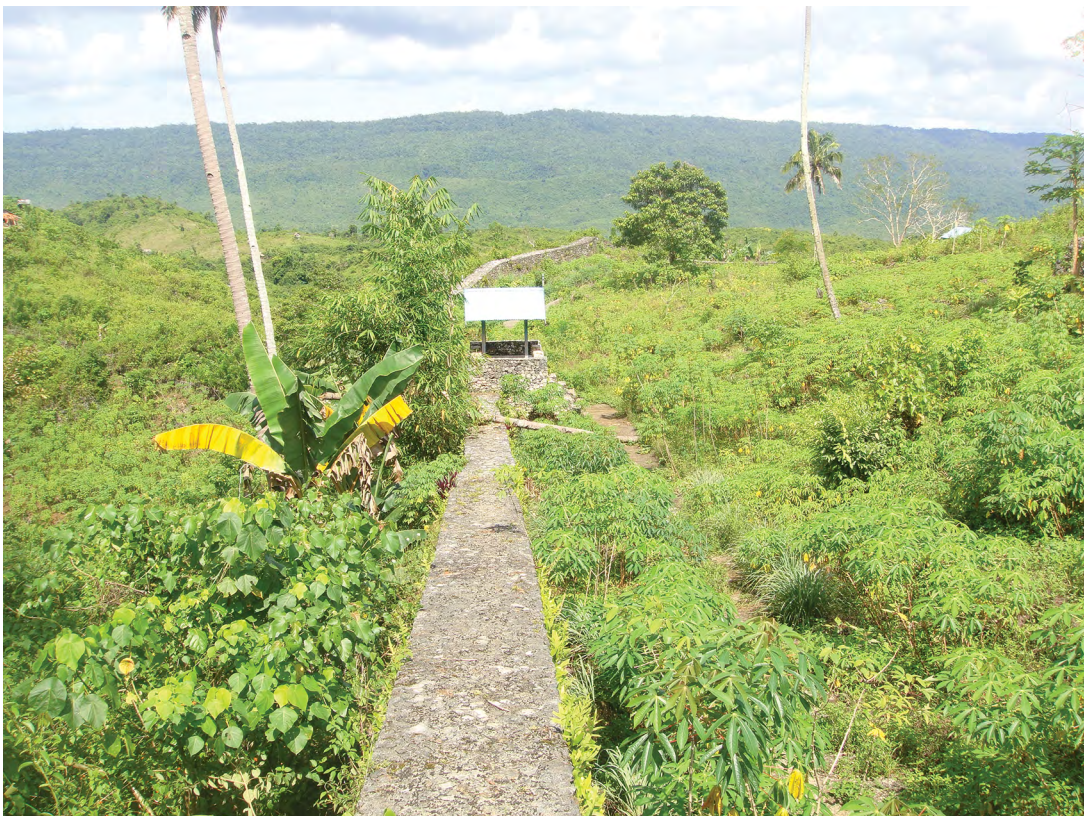
Figure 8.16. Fort Takimpo walls.
