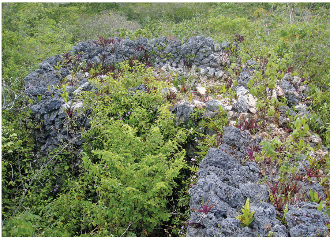
Figure 8.7. One of the corner bastions of Fort Liwu.
