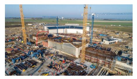
Fig. 1 ESS under construction in Lund, Sweden. The central concrete structure will house the neutron production target
