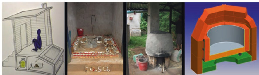
Fig. 5.7 The CaSa approach to EcoSan analysed in the present work comprises a UDDT (left) and sanitation oven (right). (Photographs by A. Krause, sketches from CaSa (2012))
