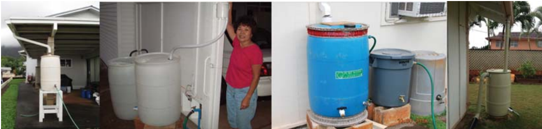
Figure 7.11 BWS' customers' testimonials and examples of rain barrel finished home installations.
