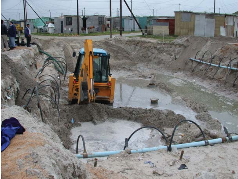
Figure 10.6 Excavating and de-watering the site for the 1065 mm chamber.
