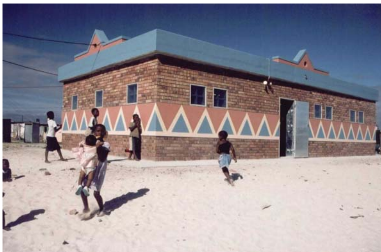
Figure 10.11 Completed chamber in Khayelitsha.
