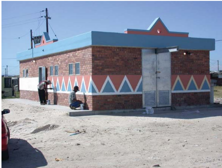
Figure 10.10 Local community painting the 1065 mm diameter chamber.
