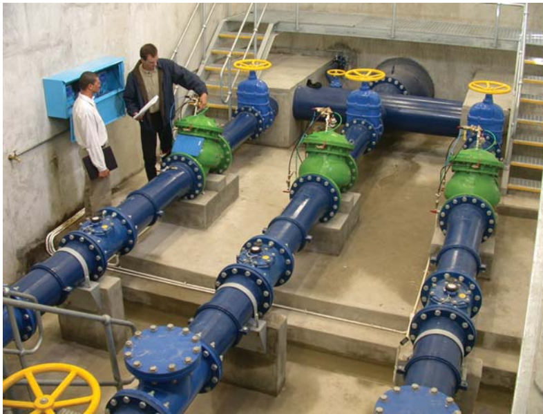
Figure 10.7 Internal view of a portion of the 1065 mm diameter chamber.
