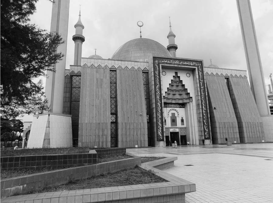
FIGURE 3.2 National Mosque in Abuja. Photo by Murtala Ibrahim.
