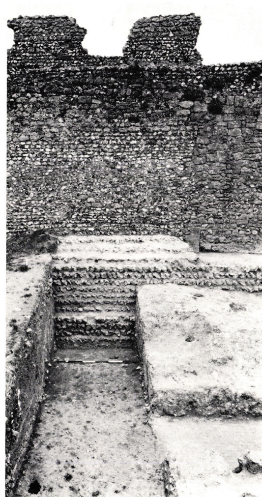
b. The internal face of the south wall exposed in trench 107 after the partial removal of the clay bank to the original ground surface (photo: Mike Rouillard)
