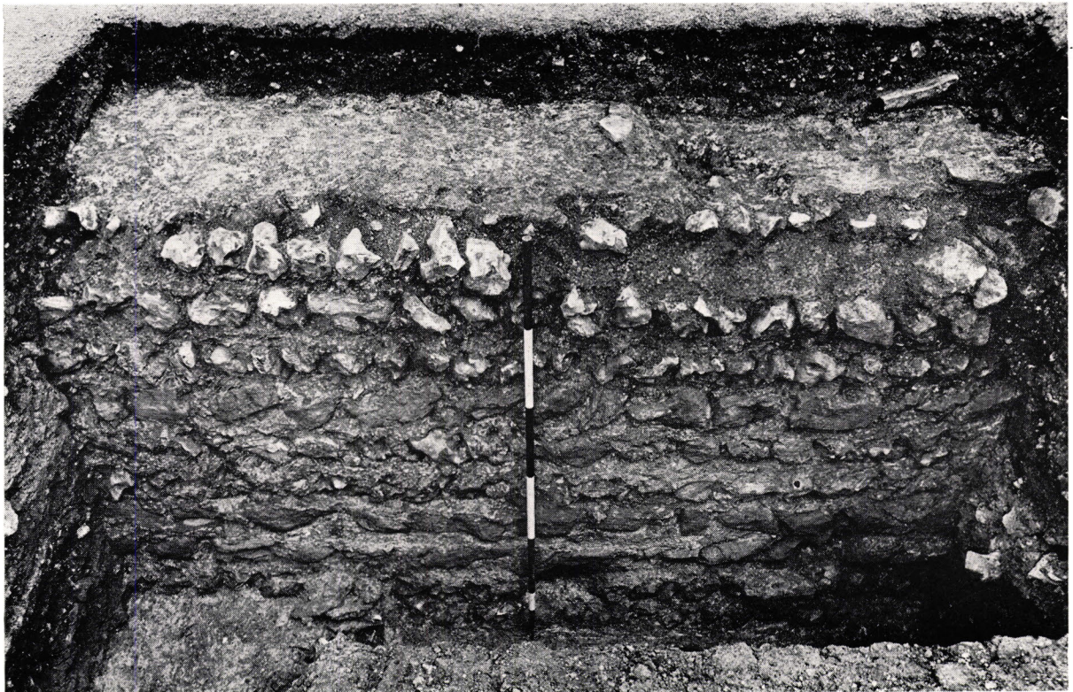
b. The watergate: the south face of the north inturned wall (photo: David Baker)
