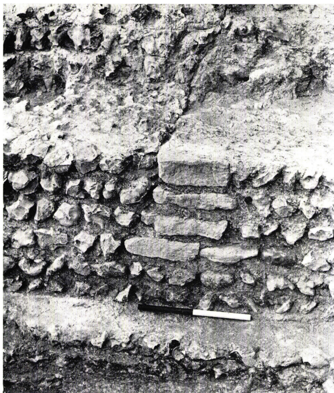
a. The west wall, as exposed in the 1961 excavation, showing the join of two working parties (photo: David Baker)
