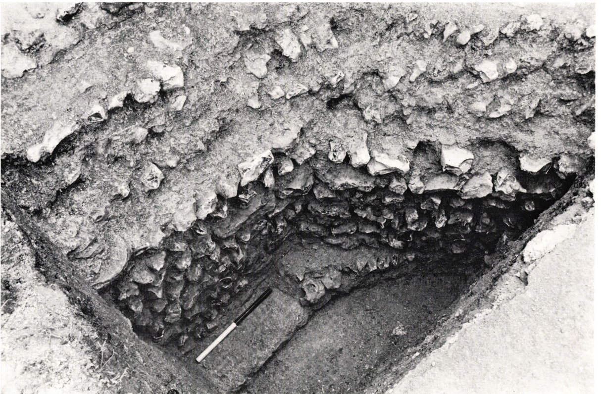
b. Bastion no. 18 showing the inner face of the fort wall behind the bastion (photo: David Baker)
