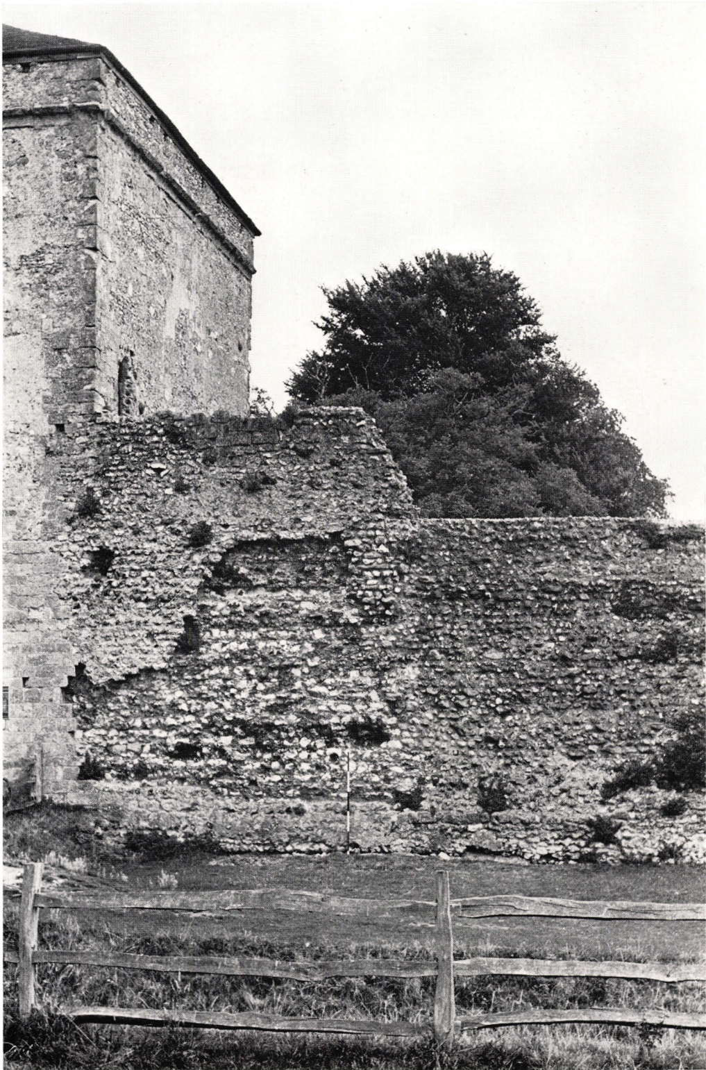
The landgate, showing the Norman blocking wall, built with chalk blocks in its core, and the adjacent Roman wall to the right of the road (photo: David Baker)
