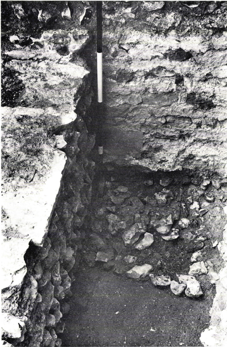
a. The landgate: inside the fort showing the junction between the Norman blocking wall (right) and the Roman gate wall. The flints are the foundation of the Norman wall (photo: David Baker)
