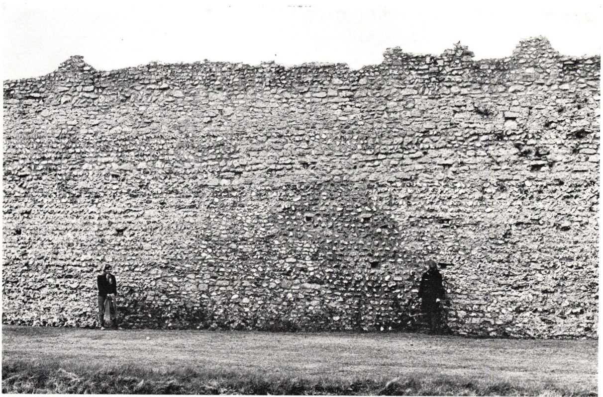
a. The site of bastion no. 7. The figure stands at the extremity of the bastion footing exposed in the excavations (photo: David Baker)
