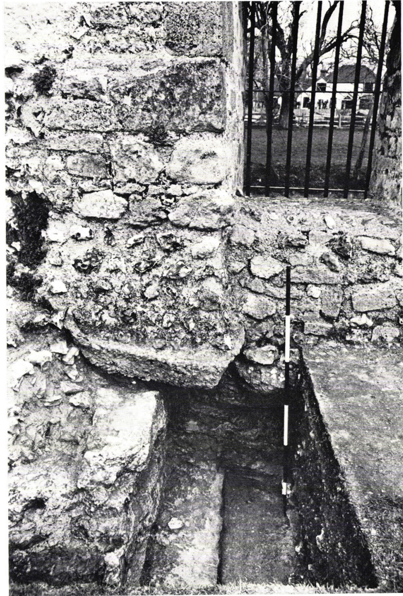
b. The north postern gate: general view showing Roman footings and the medieval gate partly underpinned (photo: David Baker)
