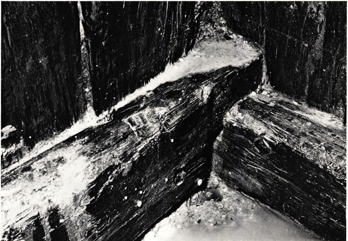
a and b . Well (pit) 135: details of the timber joints of the basal frame (Photographs: David Leigh)
