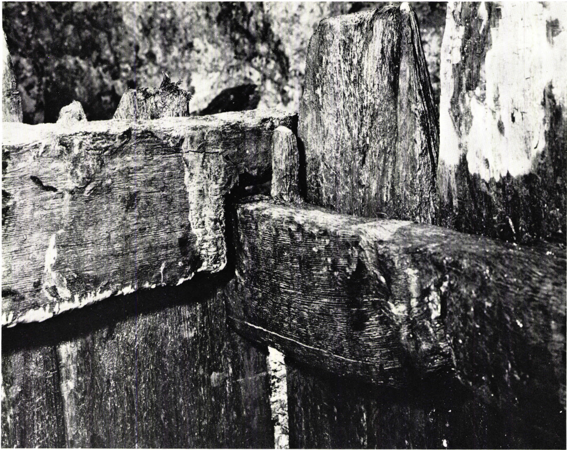
a. Well (pit) 135: detail of joint of the upper frame
