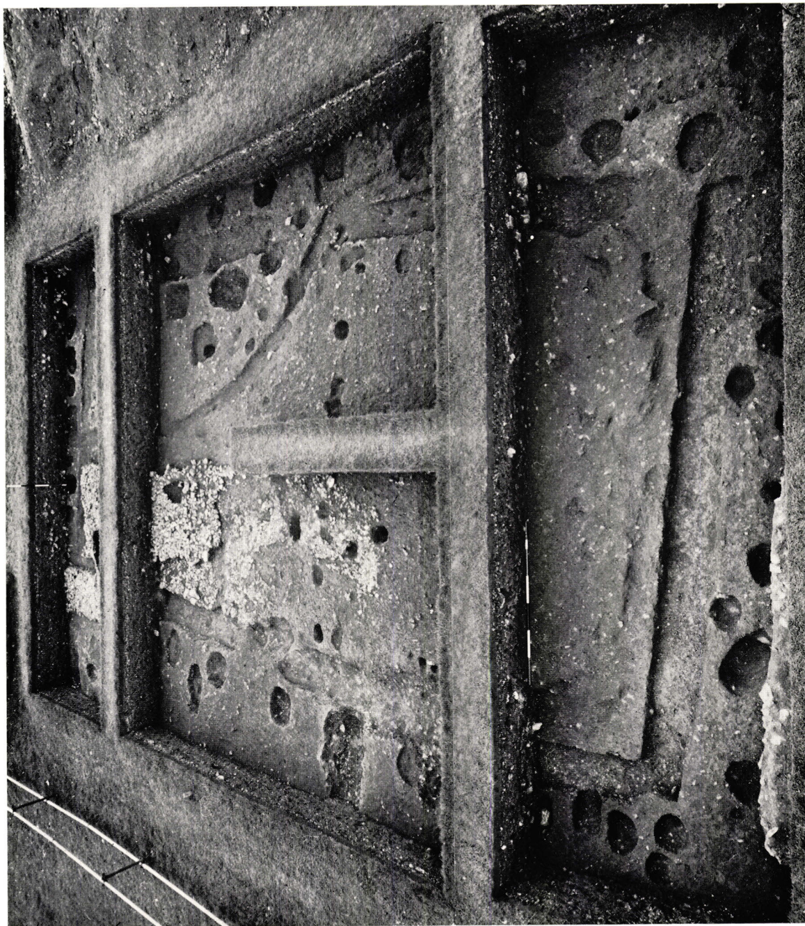
Building S13 ( Photograph: David Baker )
