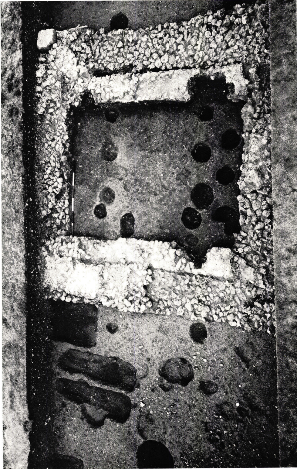
Masonry tower, building S18 ( Photograph: David Baker )
