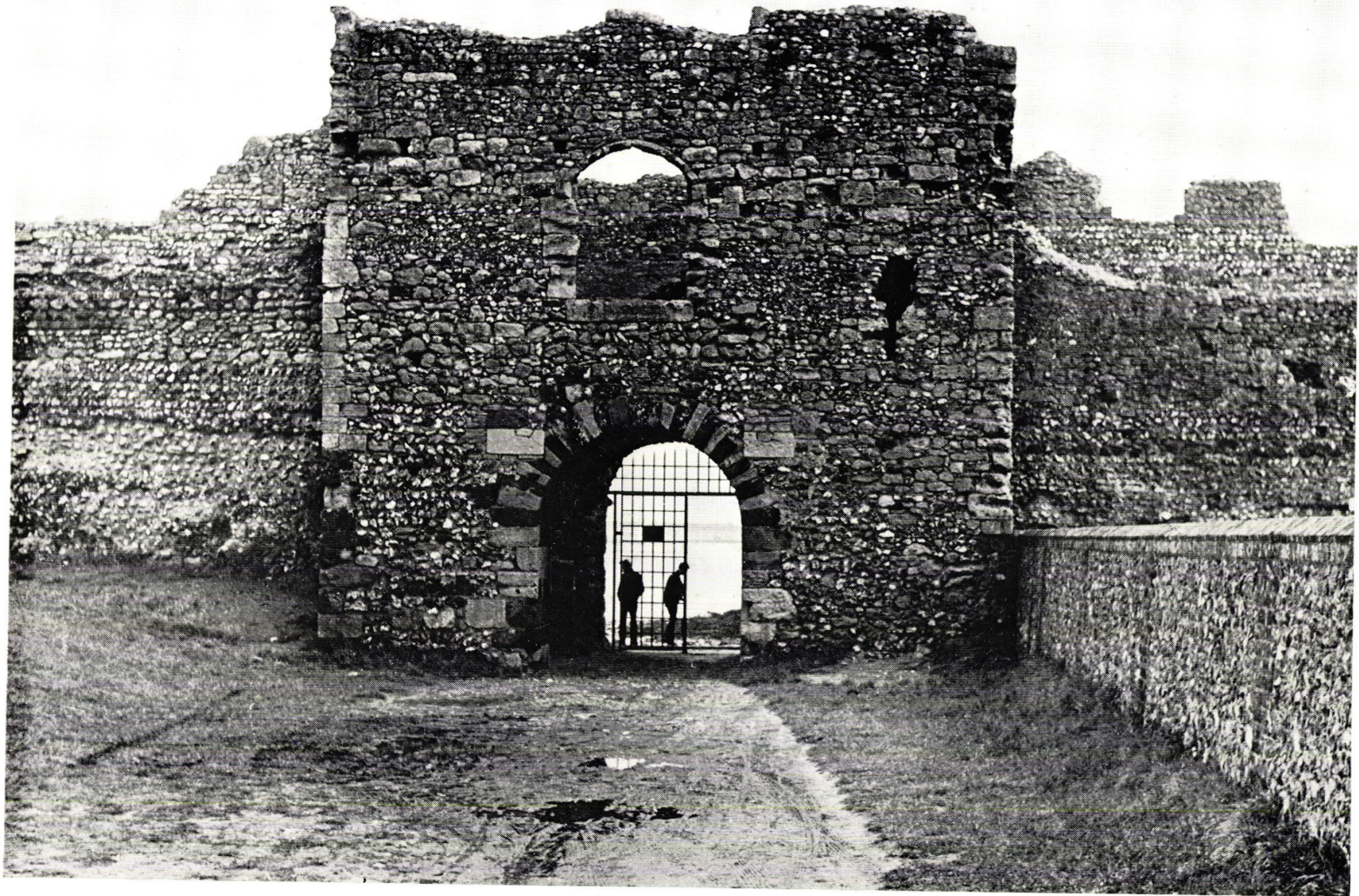
West elevation of the watergate showing eleventh-century arch with fourteenth-century rebuilding above (Photograph: David Baker)
