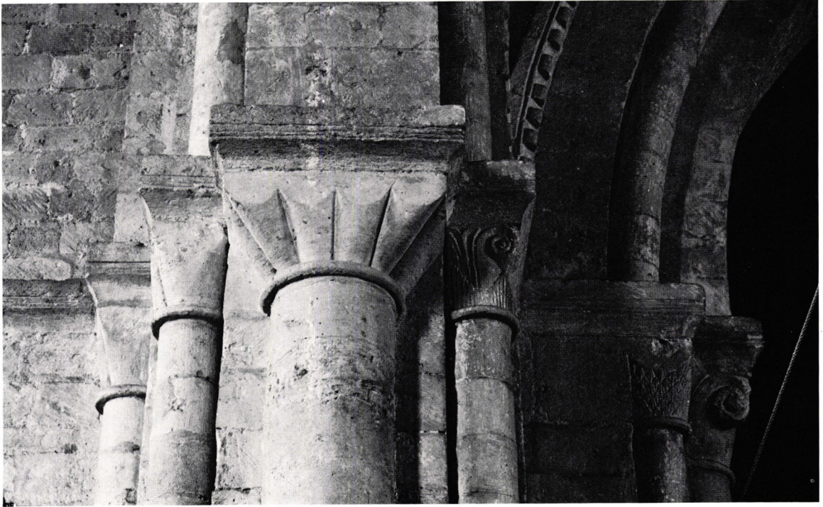
a. St. Mary's Church: capitals of north-east crossing pier, west face (photo: Mike Rouillard)
