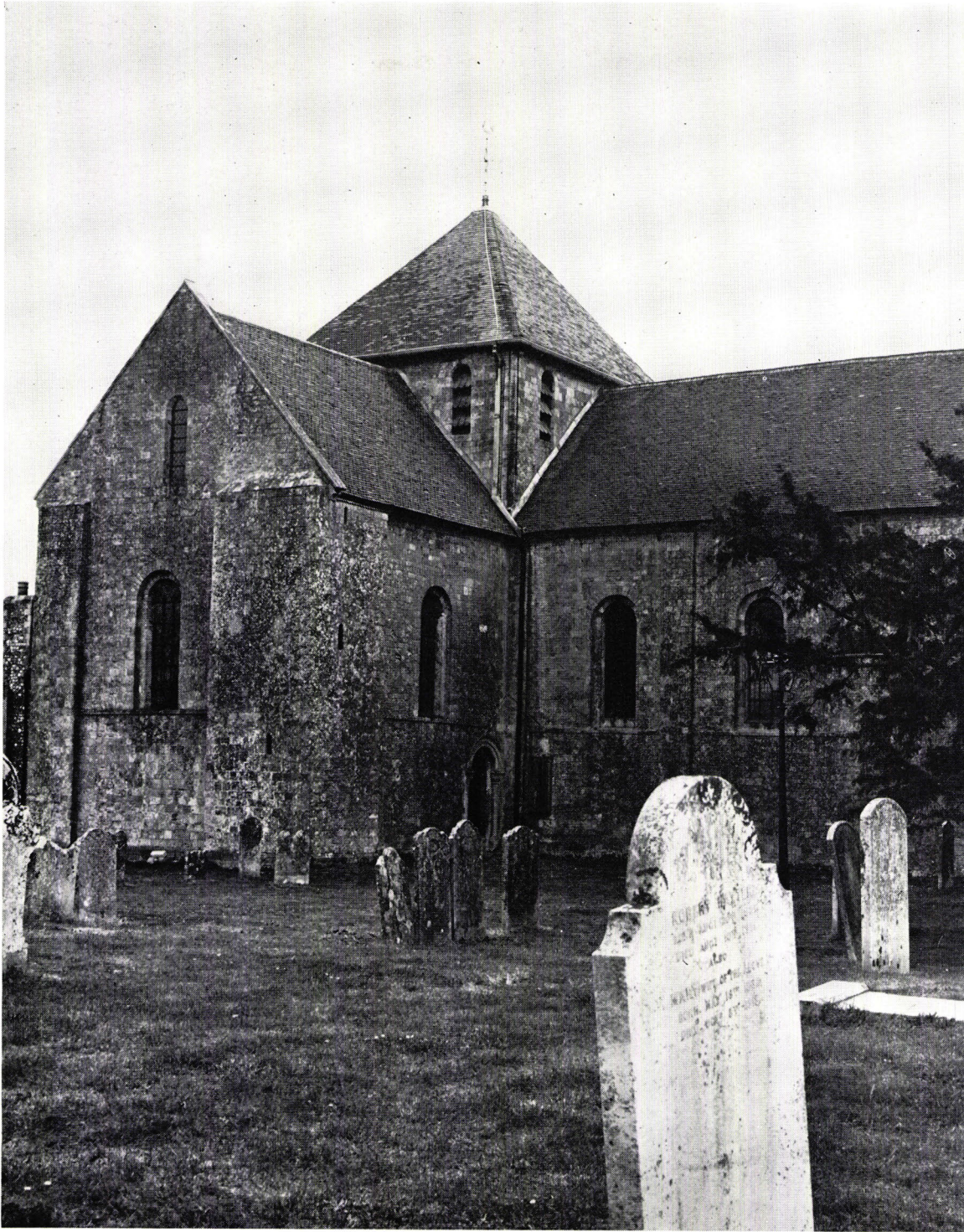
St. Mary's Church: view from the north-west (photo: Mike Rouillard)
