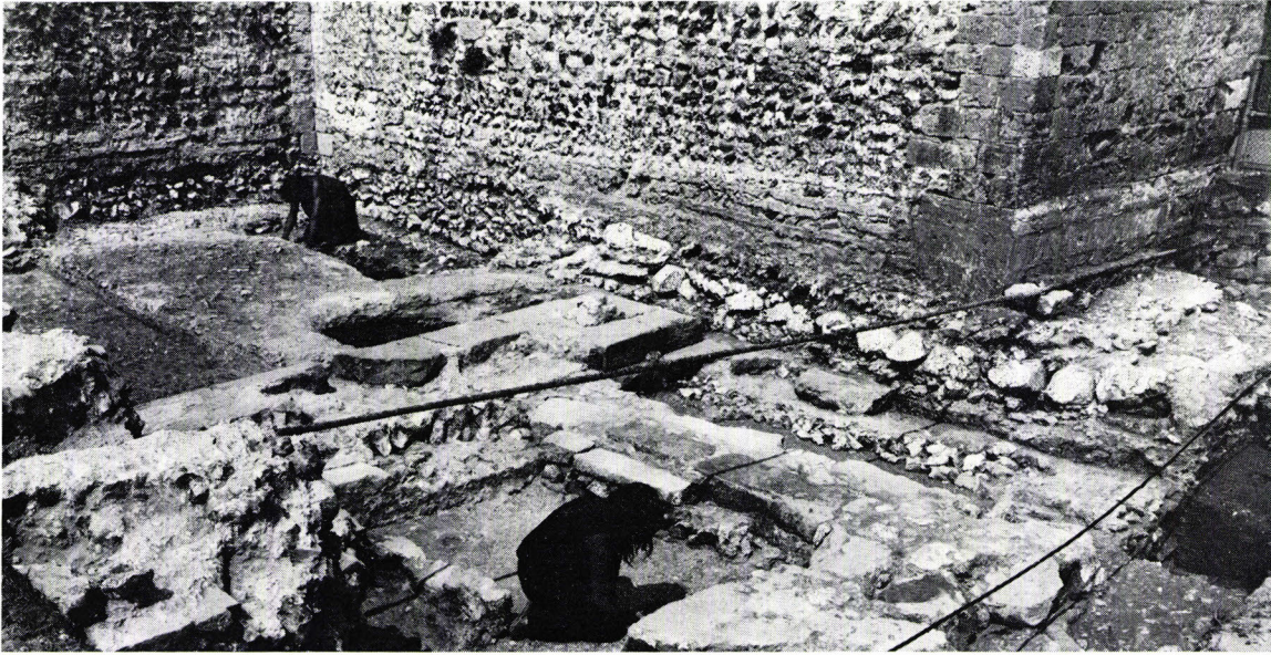
a. The landgate during excavation. Roman gatehouse in the foreground with the unweathered face of the Norman landgate beyond (photo: Mike Rouillard)
