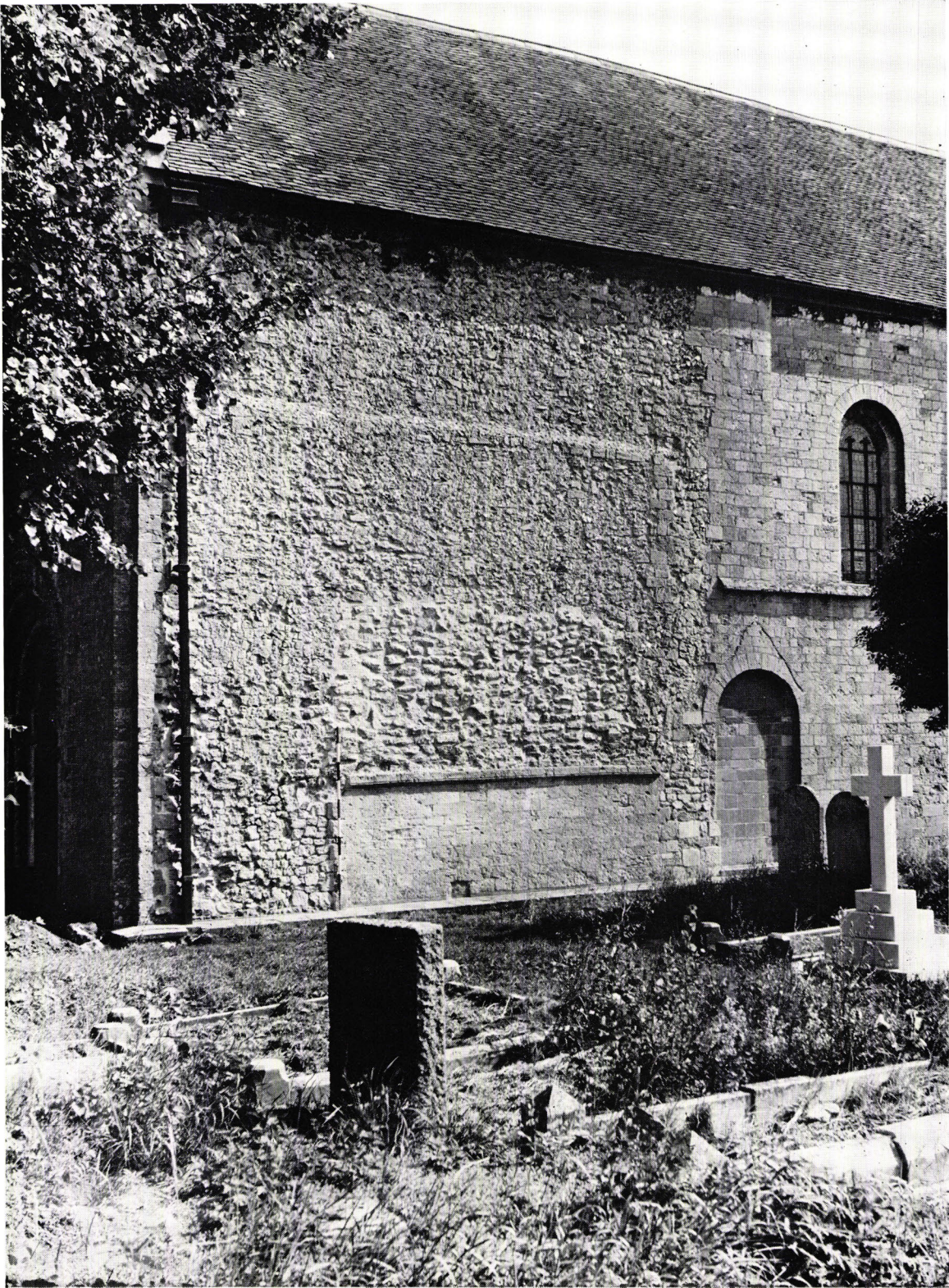
St. Mary's Church: face of south wall showing the abutment of the demolished west range (photo: David Baker)
