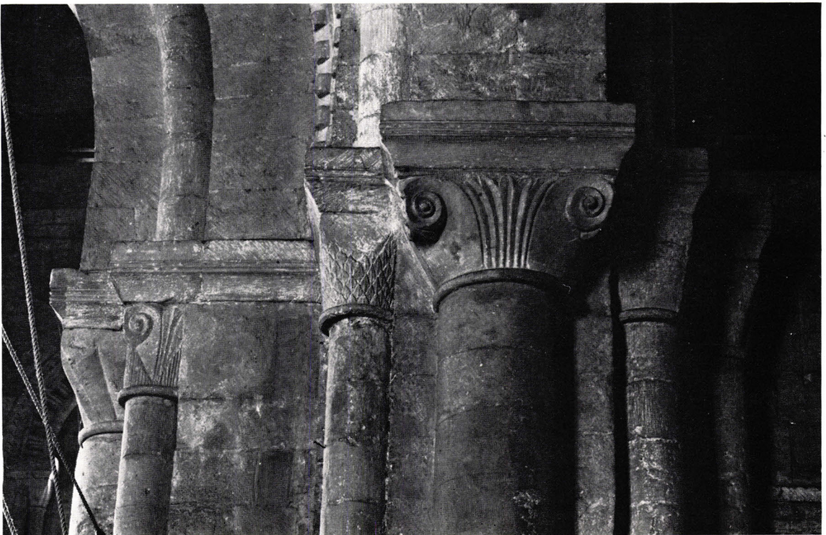
b. St. Mary's Church: capitals of northeast crossing pier, south face (photo: Mike Rouillard)
