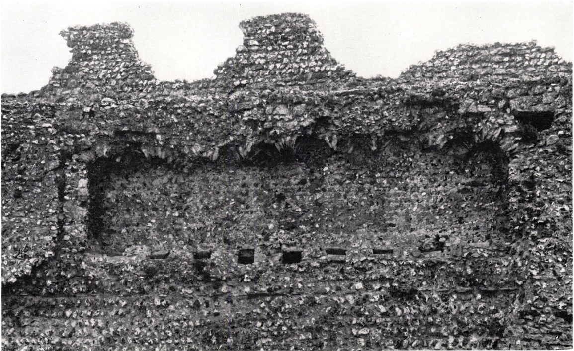
a. Priory: garderobe abutting the north face of the south wall of the Roman fort (photo: David Baker)
