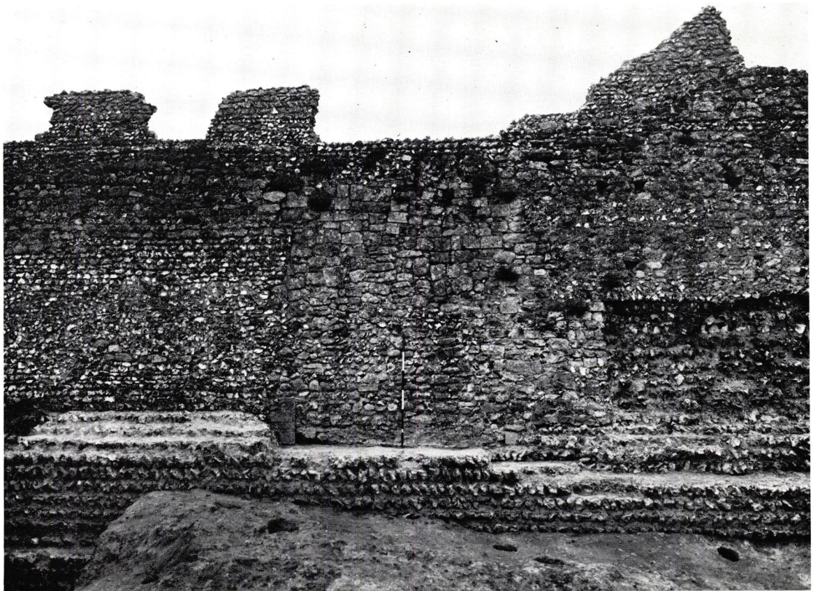
b. The medieval south postern gate, later blocked (photo: Mike Rouillard)
