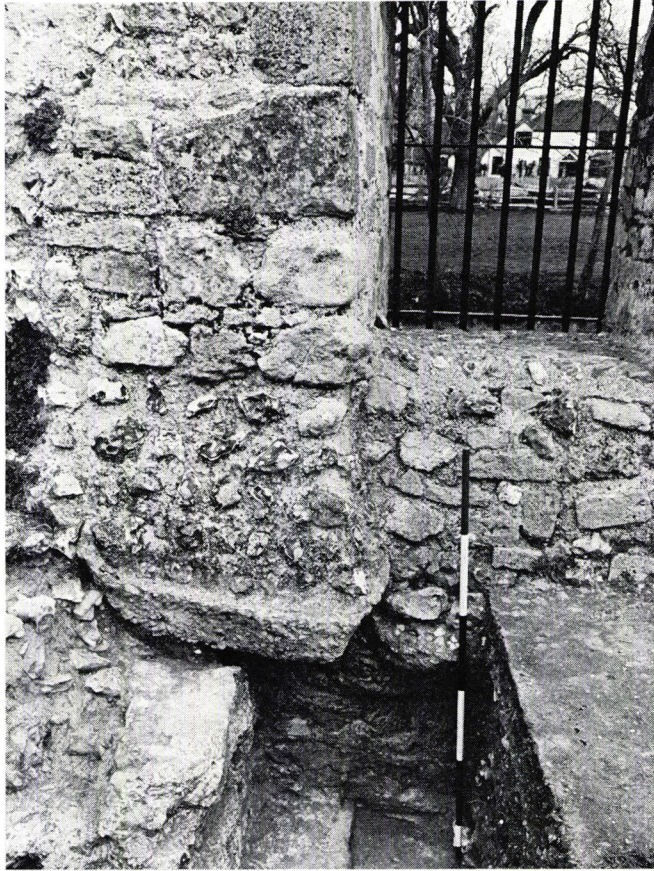
a. The Roman north postern gate blocked in the early medieval period and later re-opened (photo: David Baker)
