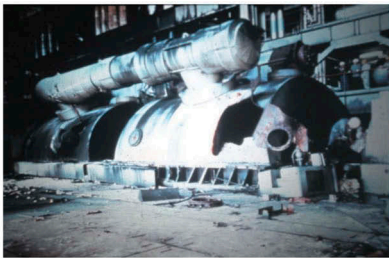
(a) Low pressure (LP) turbine casing
