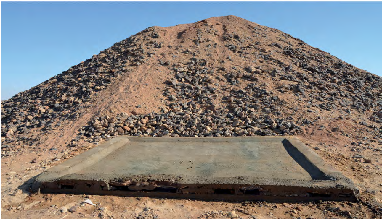
FIGURE 3.42 Tumulus 7, external shaft protected by a tin roof (top) reinforced with concrete mortar (bottom) PHOTOS BY A. KAMROWSKI [TOP], Z. KOWARSKA [BOTTOM]
