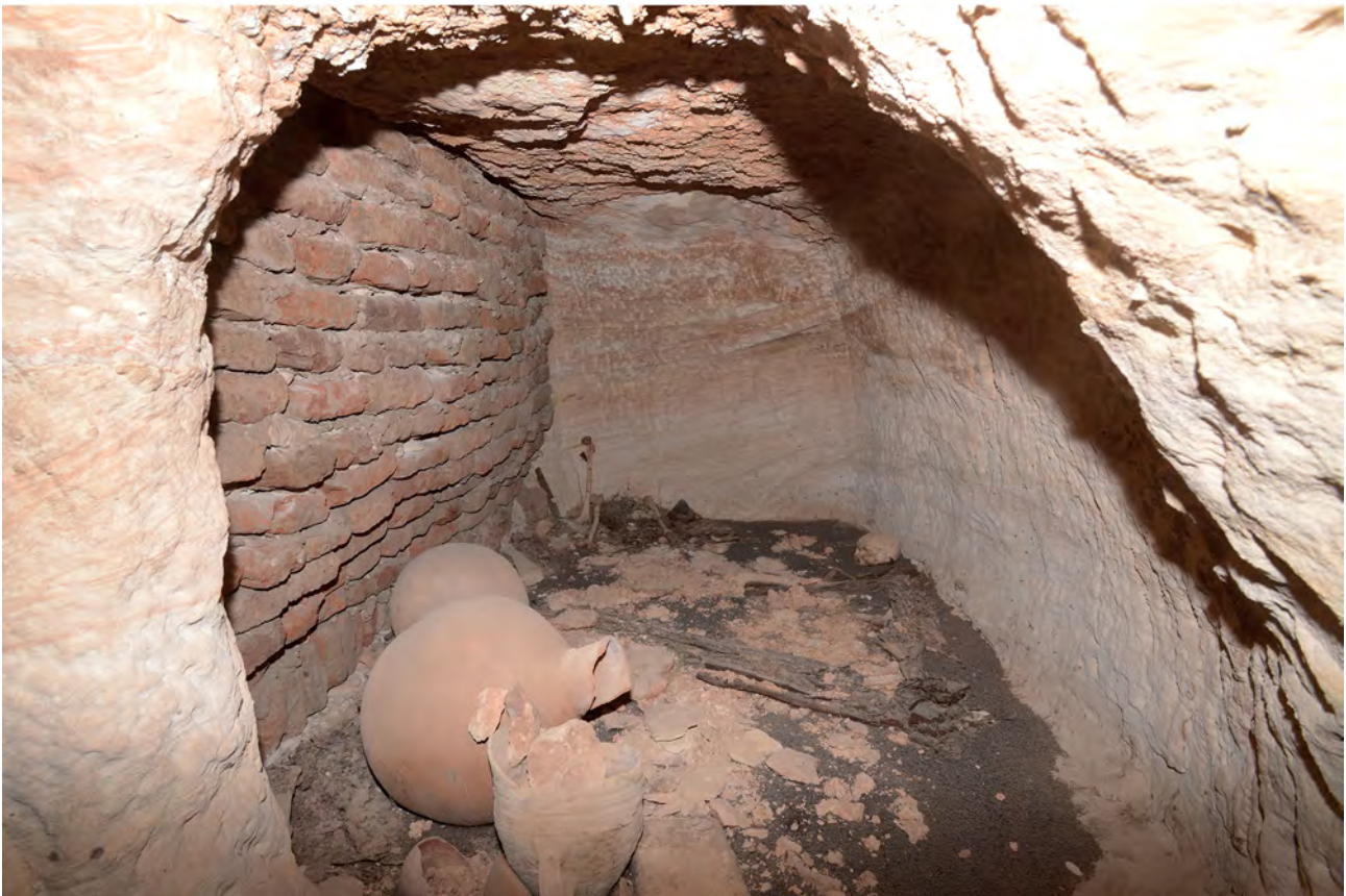
FIGURE 3.41 Tumulus 7, view of the red-brick wall on the west side of the main burial chamber—note the poor workmanship (top); east side of the burial chamber (bottom) PHOTOS BY A. KAMROWSKI
