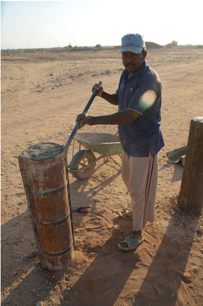
FIGURE 9.7 Construction of the concrete posts PHOTO BY A. KAMROWSKI
