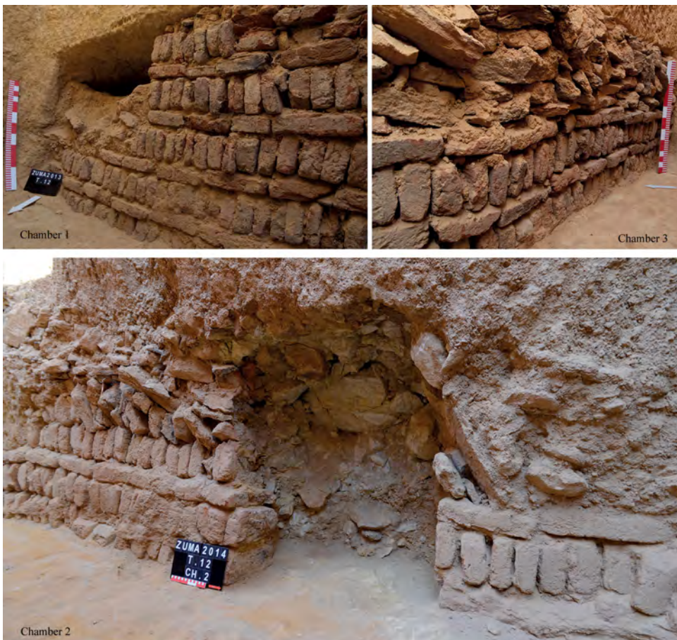
FIGURE 3.46 Tumulus 12, red-brick blocking wall in chamber 1 (top left); red-brick blocking wall in chamber 3 (top right); view of the collapsed ceiling on the north-west side of chamber 2, facing west (bottom) PHOTOS BY E. SKOWROŃSKA
