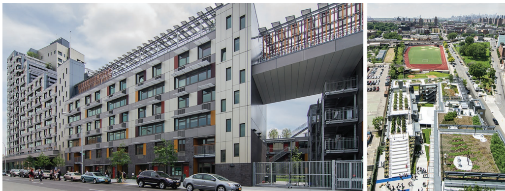
FIGURE 11.3 Via Verde Sustainable Mixed-Income Housing in New York City. Source: New York City Housing Development Corporation.
