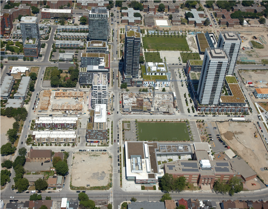
FIGURE 10.2 Regent Park Phase Two Development.
