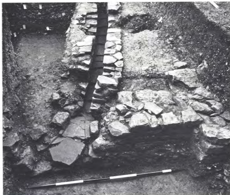
(b) the drain passing through the east wall of the building; looking west
