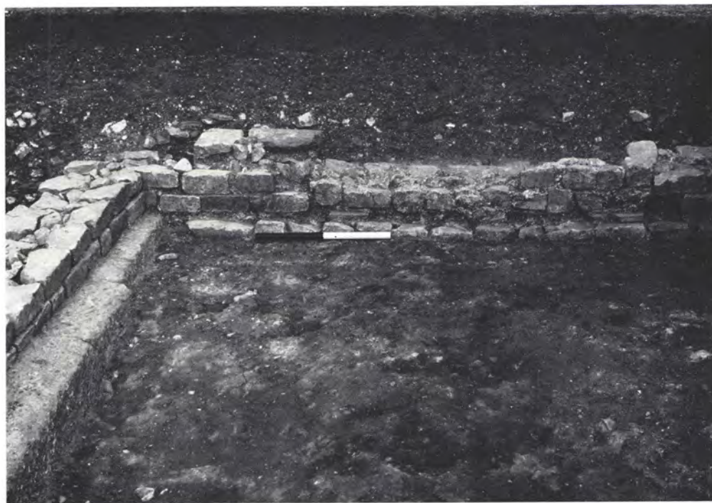
b. Room B of the East Wing baths showing the blocked door in the east wall; looking east (p. 173)
