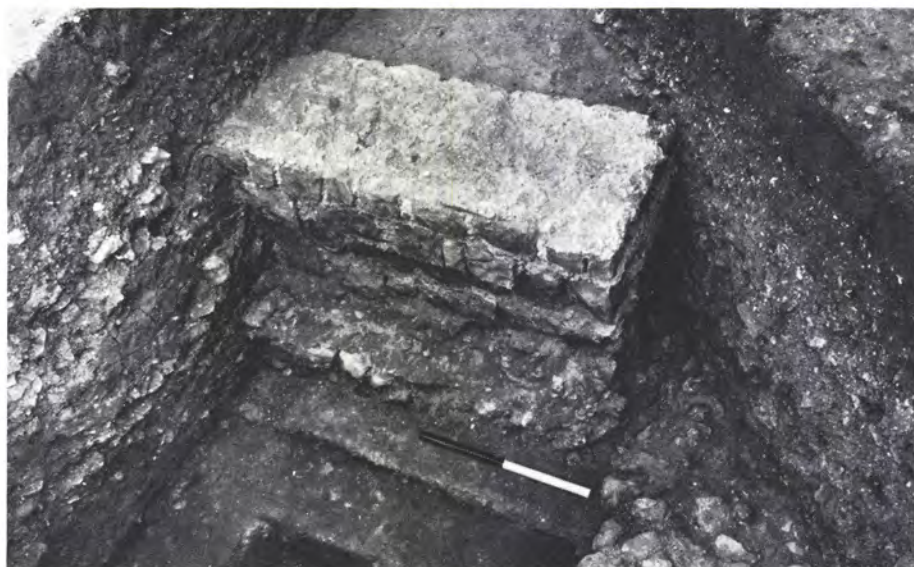
a. North wall of room E 9 showing ashlar masonry partly off the line of the flint footings; looking north (p. 82)
