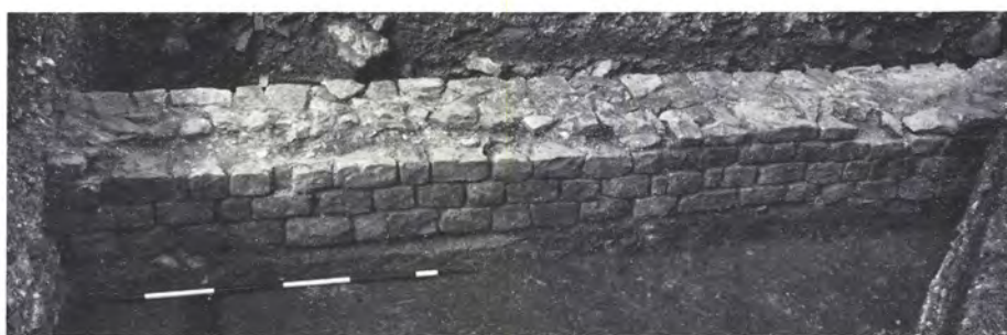
c. East wall of East Wing opposite rooms E 9 and 11; looking west (p. 82)
