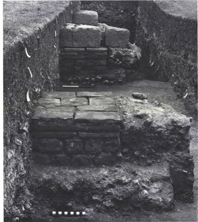
b. The Aisled Hall showing the structure of the original pier bases with their later additions; looking west (p. 106)
