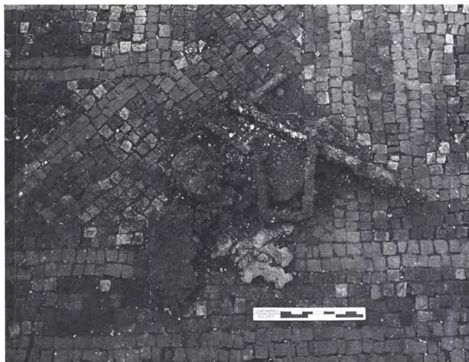
b. Lead puddle and collapsed iron work on the floor of room N 12; looking east (p. 188)
