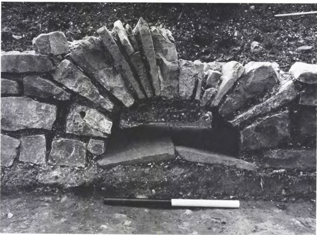
b. Tile and greensand arch through the east wall of the East Wing; looking west (p. 134)
