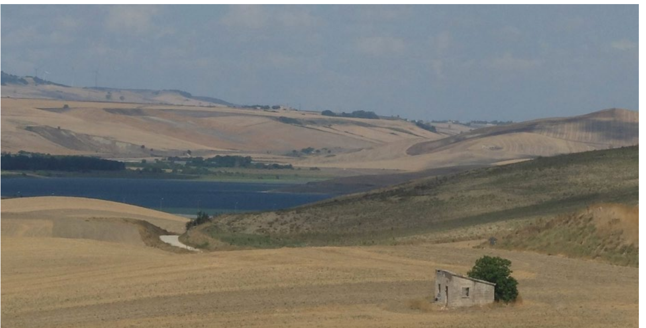
Photo Overview-2. The reservoir created by the Basentello dam, seen from near Vagnari.
