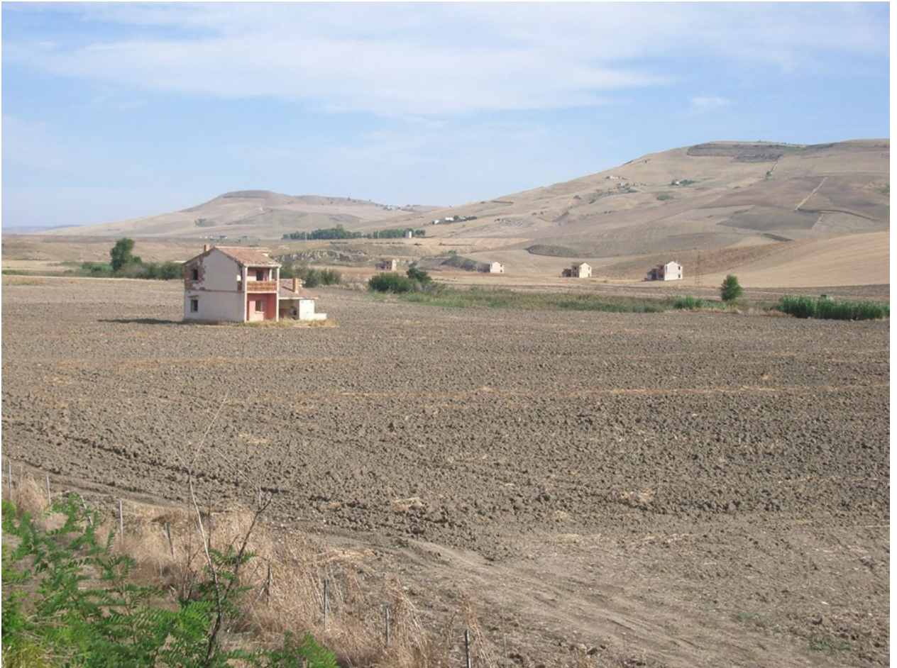
Photo Overview-1. Abandoned reform houses of the fascist period on the alluvial fill beside the Basentello.
