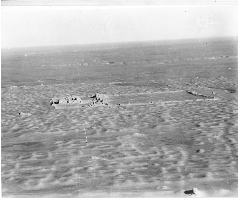
Figure 1: Aerial view of the city of Hatra from south (RAF '30s).
