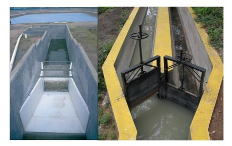
**Figure 9.9** Left: A properly installed, prefabricated Parshall flume used to measure influent flowrates to a facultative pond. Accurate flow measurement is essential for assessment of hydraulic and organic loadings to the pond system. Right: Well-designed and installed sluice gates in a dual channel grit chamber; the gates have metal-to-metal contact that are routinely greased for ease of operation (left photo: El Paraíso, Honduras; right photo: Suchitoto, El Salvador).
