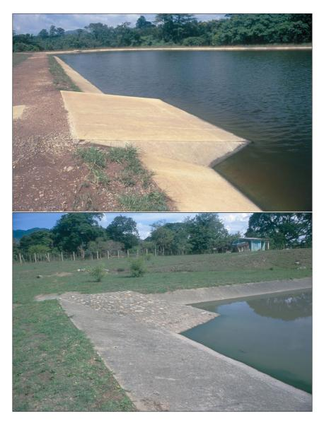
**Figure 9.29** Examples of access ramps for sludge removal in primary ponds. Top photo: facultative pond, Santa Cruz de Yojoa, Honduras. Bottom photo: anaerobic pond, Danlí, Honduras.
