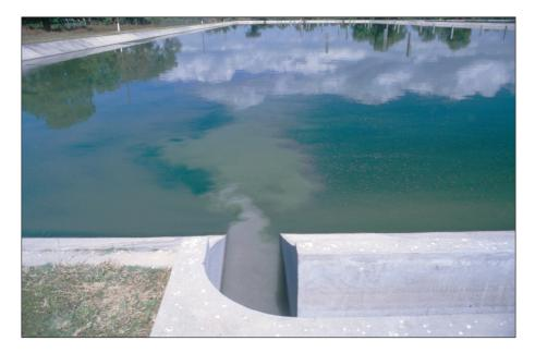
Figure 9.12 A good example of an inlet structure with open channel that enters this facultative pond at the water level. The raw wastewater plume entering the pond is clearly seen to be approximating plug flow (Granada, Nicaragua).
