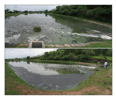
**Figure 5.21** Single inlets in facultative ponds such as this one cause sludge accumulation immediately downstream of the inlet. The sludge accumulation in turn diverts inflow, forming preferential flow paths and dead zones, reducing the hydraulic efficiency of the pond (Zaragoza, El Salvador).
