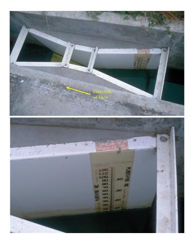
**Figure 4.11** An example of a pre-fabricated Parshall flume installed for a horizontal flow grit chamber. The designer should always specify pre-fabricated and calibrated Parshall flumes in the design to avoid the construction problems shown in Figures 4.13 and 4.14 (Masaya, Nicaragua).
