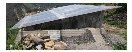
**Figure 8.8** The existing reservoir at the San Antonio, Sololá wastewater reuse project has an estimated maximum volume of 50 m<sup>3</sup> and was designed for a pilot irrigation project of 1.84 ha.
