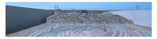
**Figure 6.17** Rock Filter 1 under construction. The three filters in parallel were designed for a water depth of 2.0 m, with 0.2 m of filter above the water surface, with a design  $HLR_{filter} = 0.15 \text{ m}^3/\text{m}^3 \text{ d}$ . See also Figure 6.6.
