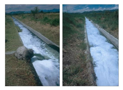
**Figure 9.22** An example of the foam that can be formed by turbulence when the final discharge is above the water level in the receiving canal. Foam is caused by detergents and other non-biodegradable surfactants in wastewater. The way to control foam production is to use subsurface discharge devices as shown in Figure 9.21 (Villanueva, Honduras).
