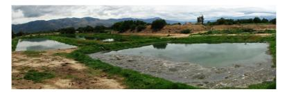
**Figure 1.26** An abandoned waste stabilization pond system in Tarata, Bolivia. The effluent discharges to a small river used for irrigation by farmers (indirect reuse). The health risks are high for farmers, their families, and the consumers of produce. Waste stabilization ponds are the recommended system for treatment and reuse in agriculture, but even the most appropriate, sustainable technologies require operation and maintenance.
