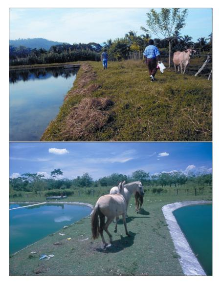
**Figure 9.30** The area encompassing the entire stabilization pond system should be fenced, preferably with barbed wire, to prevent the entry of animals, which can damage embankment slopes and serve as sources of infection, and that of unauthorized persons (photo above: Tela, Honduras; photo below: Choloma, Honduras).
