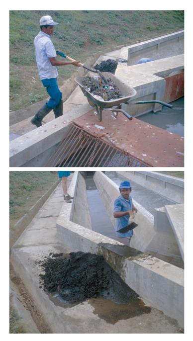
**Figure 10.1** In preliminary treatment, the operator's responsibility is to clean the bar screen daily, and the grit chamber when needed – typically once a week in small systems. It is essential to agitate the settled solids in operating grit chamber on a daily basis so that entrapped organic solids escape to the downstream pond, and inorganic solids remain in the channel. The solids from the bar screen and grit chamber should be buried and covered on a daily basis (Leon, Nicaragua).
