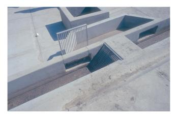
**Figure 4.6** The approach channel to the bar screen should have a bypass as shown above to divert the flow during an emergency when the operator is not available to clean the screen. Note in the photo that the bars are made of aluminum. The influent bar screen should have a drainage platform as shown in Figure 4.4 (Sanarate, Guatemala).
