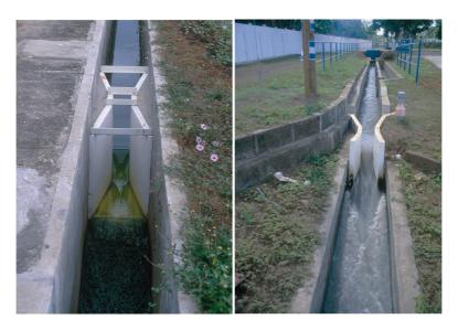
**Figure 4.12** Examples of free-flow Parshall flumes used with horizontal grit chambers. To ensure free flow, the downstream head at the maximum flowrate,  $H_{b,max}$ , must be  $\leq 0.60 H_{max}$ . In the examples above the invert elevations of the downstream canals are much lower than the Parshall flume invert and thus give an added safety factor  $(H_{b,max} \ll 0.60 H_{max})$  (left photo: León, Nicaragua; right: Masaya, Nicaragua).
