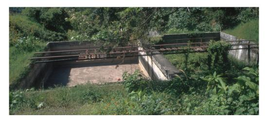
**Figure 2.8** An abandoned activated sludge treatment plant in an urbanization within the city of San Salvador, El Salvador. New developments often require wastewater treatment to be approved, and activated sludge is chosen to save land area for more housing. The cost of operation and need for skilled personnel, however, is normally beyond the resources of the urbanization, and treatment plants like this one quickly fail, if they were ever in operation to begin with.
