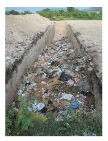
**Figure 4.18** Municipal solid waste is deposited in this trench at Villanueva, Honduras. When full, the trench is backfilled and excess soil is used for other purposes onsite. The same procedure can be used at larger wastewater treatment facilities for preliminary treatment solids and should be included in the original design of the system.
