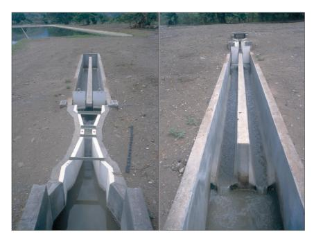
**Figure 9.8** This grit chamber was built without drainage, without sluice gates for the downstream channels, and without a Parshall flume at the outlet to control horizontal velocity. The prefabricated Parshall flume was installed on the upstream instead of the downstream end of the grit chamber! This case is typical of problems encountered with inadequate design and construction supervision (Trinidad, Honduras).
