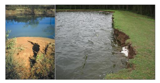
**Figure 9.3** Stormwater runoff has to be controlled to protect the interior embankment slopes of ponds. Left: In this maturation pond, stormwater runoff was not controlled and caused serious erosion to the interior embankment, which did not have protection with a revetment (Zaragoza, El Salvador). Right: Wave action driven by strong winds erodes the unprotected interior embankment of this maturation pond (Santa Cruz, Bolivia).
