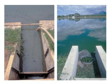
**Figure 10.6** Left photo: the outlet of a facultative pond designed with a bottom sluice gate and a rectangular weir did not have the sluice gate in place; as a result, the floating solids were carried out with the effluent over the rectangular weir, and the removal efficiency of fecal coliforms was low (Catacamas, Honduras). Right photo: a circular baffle is used to control the discharge of scum in the effluent of a facultative pond (Chinendega, Nicaragua).
