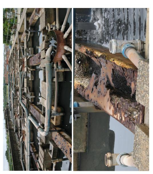
**Figure 2.14** Serious corrosion problems can arise with the production of  $H_2S$  and  $H_2SO_4$  in UASBs as shown in this unit in Aracaju, Brazil. Raw wastewater monitoring for sulfate concentrations, and the use of corrosion-resistant materials throughout the UASB, must be specified by design engineers to avoid these problems.
