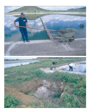
**Figure 10.5** Floating scum and solids accumulate in corners, where the operator can easily remove them with a scum rake and put them in a wheelbarrow. Afterwards, they must be buried, or covered with a layer of soil or lime. In the photo below the operators put the collected scum solids in a small excavation and cover them with lime to control odors. When the excavation is filled, it is covered with a layer of soil (Masaya, Nicaragua).
