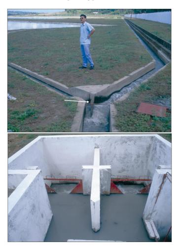
**Figure 9.16** Examples of flow distribution devices between batteries of two facultative ponds in parallel. In the top photo (Masaya, Nicaragua), an adjustable partition is used (arrow). In the bottom photo (Granada, Nicaragua), a fixed partition between ponds in the center is combined with adjustable triangular weirs. The flows to each pond must be monitored to ensure equal distribution.
