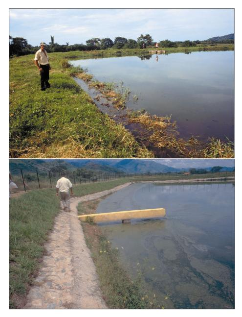
**Figure 9.26** In the photo above (Tela, Honduras), the facultative pond has serious problems with the growth of aquatic plants at the shoreline due to lack of a revetment. In the photo below (Catacamas, Honduras), the poor construction of the revetment (note the contour lines at the water level) with insufficient freeboard does not prevent the growth of aquatic plants.
