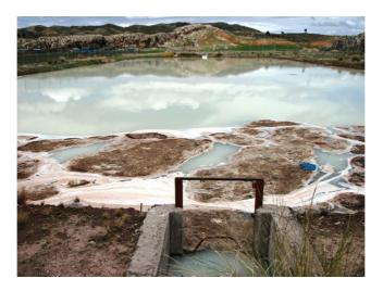
**Figure 3.2** A facultative pond receiving domestic wastewater from the municipality of Huata, Peru (Population  $\sim$ 1600) overloaded by discharges of cheese processing wastewaters. In this case, a small cheese processing plant had much stronger wastewater than the design population.
