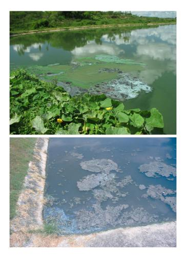
**Figure 10.3** Scum, floating solids, and aquatic plants usually accumulate in the corners of ponds, driven by winds. An operator needs a scum rake and a wheelbarrow to remove these solids. If the solids are not removed frequently, they will emit odors due to decomposition and serve as suitable foci for the attraction and reproduction of insects (top photo: Lagartos, Brazil; bottom photo: Villanueva, Honduras).
