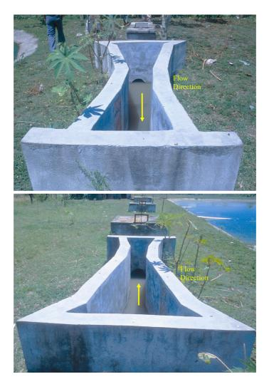
**Figure 4.14** Another example of a poorly designed and constructed Parshall flume without free-flow (Choloma, Honduras). Pre-fabricated Parshall flumes are always recommended to avoid this common problem.
