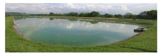
**Figure 6.8** An unbaffled maturation pond with l/w = 5.4/1 (285 m × 53 m), with the inlet at the water surface. Short-circuiting is not apparent, but monitoring data are not available and performance cannot be assessed, a common problem. (Choloma, Honduras).
