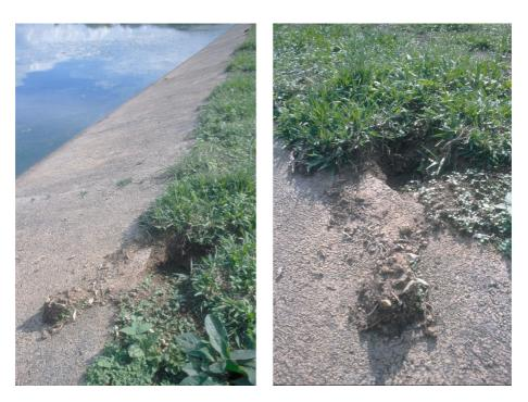
**Figure 10.11** Turtle excavations behind the revetment in a secondary facultative pond. Turtles can burrow behind and under geomembrane liners and the revetment to deposit their eggs. The operator should monitor the condition of a liner and revetment routinely when there are high turtle populations in the ponds (Danlí, Honduras).
