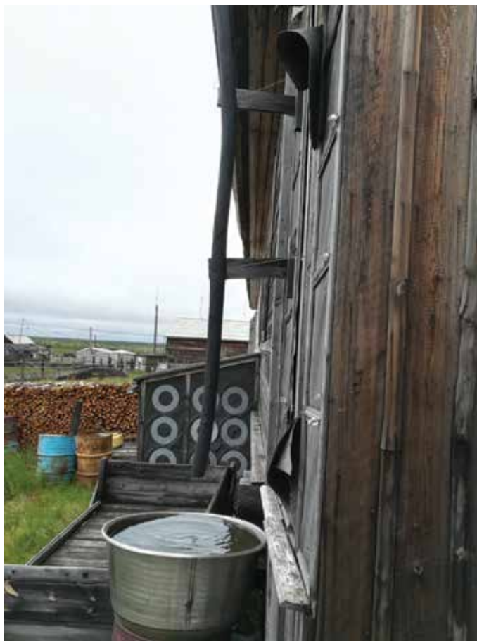
Figure 12. Rainwater harvesting for personal consumption, Khayyr (even community), Ust-Yanskiy region, Yakutia (photo: V. Gassiy).
