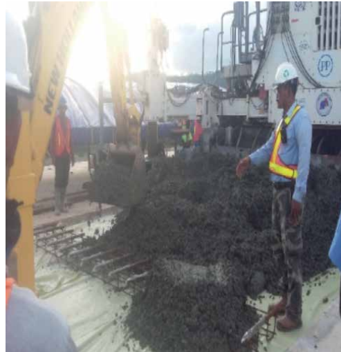
Figure 10. Pouring, flattening, and layering of the concrete/rigid pavement. Compaction process.
