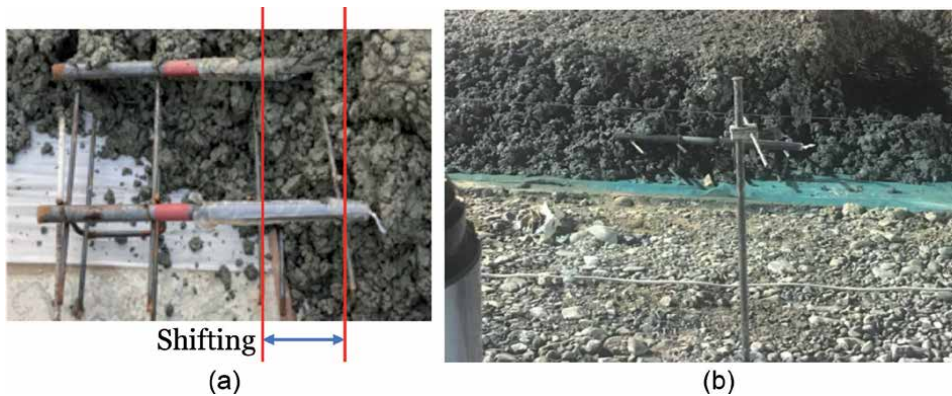
Figure 11. Shifting dowel: (a) the top dowel holder shifts, and (b) the dowel holder shifts.
