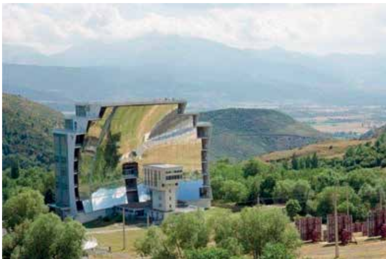
Figure 1. General view of the France furnace.
