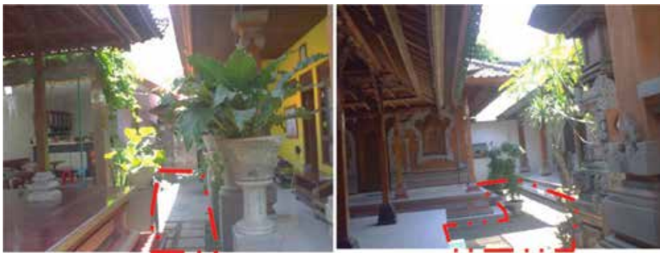
Figure 4. Courtyards ( natah ) that have been changed.
