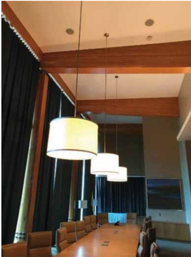
Figure 6. Conference room built with GLT beams and columns at the University of New Brunswick, Fredericton, Canada.
