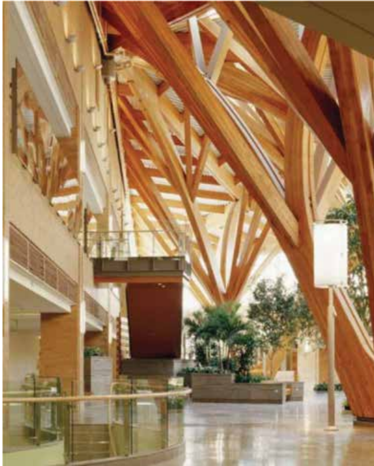
Figure 7. A forest of intertwined GLT trees in the Carlo Fidani Peel Regional Cancer Centre, Mississauga, Canada (Source: Photos obtained from CWC [12]).
