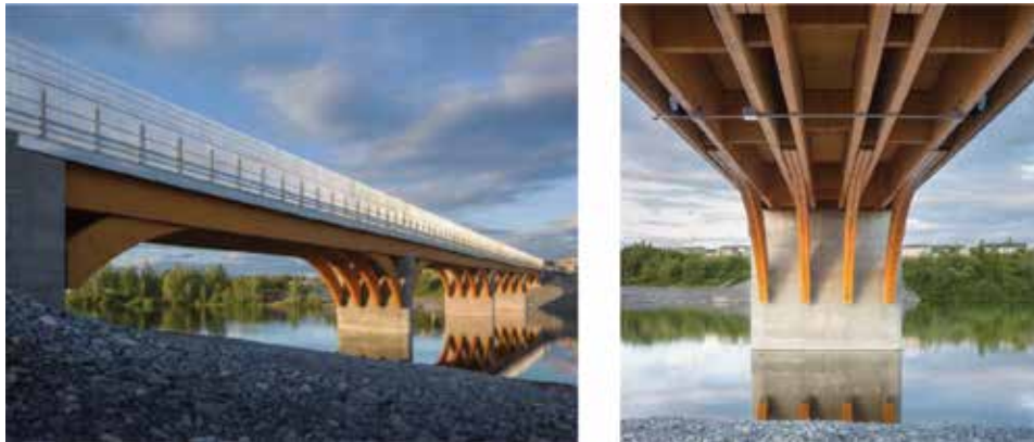
Figure 8. 160-m-long timber bridge with GLT deck structure in Mistissini, Canada. (Source: Photos obtained from Lefebvre and Richard [13]).
