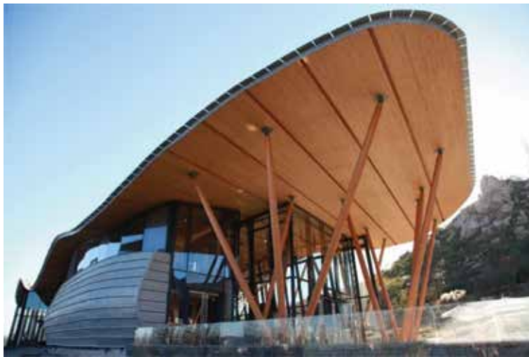
Figure 12. Qingdao Pearl Visitor Centre of exposed NLT roof in China (Source: Photo obtained from StructureCraft [16]).
