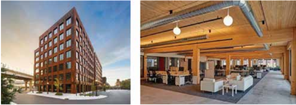
Figure 11. Seven-story T3 Minneapolis building made of NLT floors and GLT beams and columns in USA (Source: Photos obtained from StructureCraft [16]).
