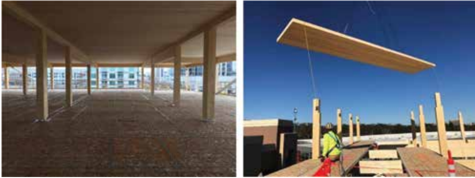
Figure 15. Seven-story T3 Atlanta building comprising DLT floor and roof panels in USA (Source: Photos obtained from StructureCraft [18]).
