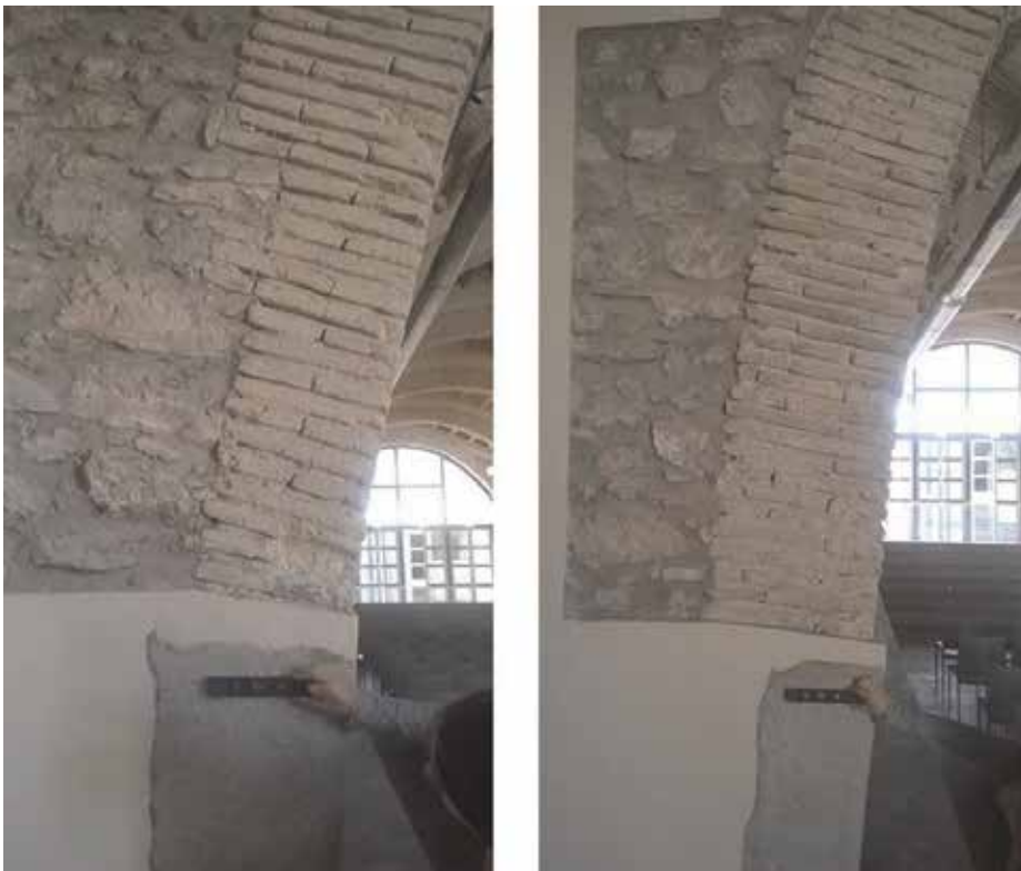
Figure 21. Springing of arches no. 1 and no. 2 in the O'Connor cellar.
