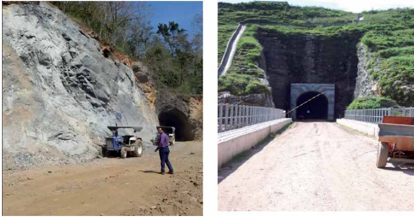
Figure 5. View of approaches to the tunnel constructed in the hill.
