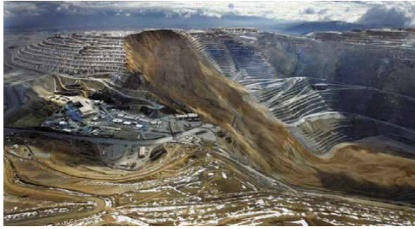
Figure 25. Circular slope failure at the open pit of the Bingham Canyon Mine in Utah.
