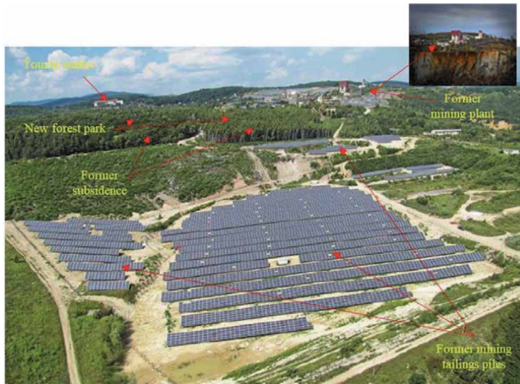
Figure 6. The subsidence of Košice-Bankov after reclamation; panoramic view—Summer 2016. Solar collectors on the places of the former mining tailing piles; new forest park in the background on the places of the former subsidence.
