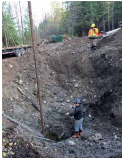
Figure 9. Views of site E with wood crib within the shoreline forest of Smith's Bay. Figure is from November 1, 2016, and shows the excavation in progress with the discovery of a barrel at ~5 m below grade but still 4 m above the well box [21].
