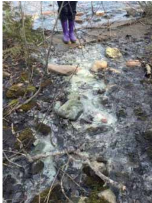
Figure 12. Views of site F. Figure shows the seepage path from site F to the lake on April 29, 2016, with white foam arising from the wooden crib.
