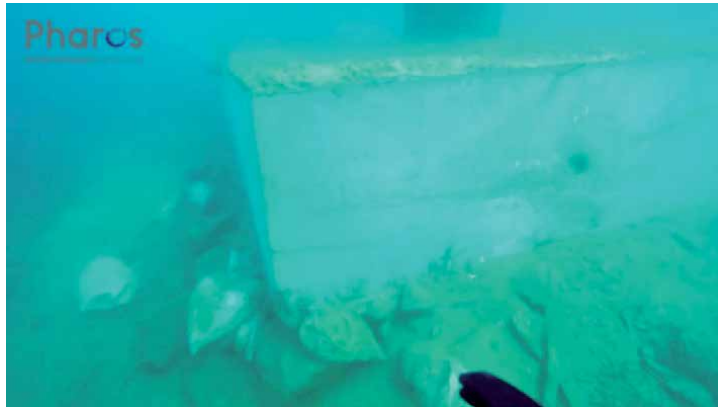
Figure 25. Corner detail of the Duke of Alba's foundation slab (Port of Naos).
