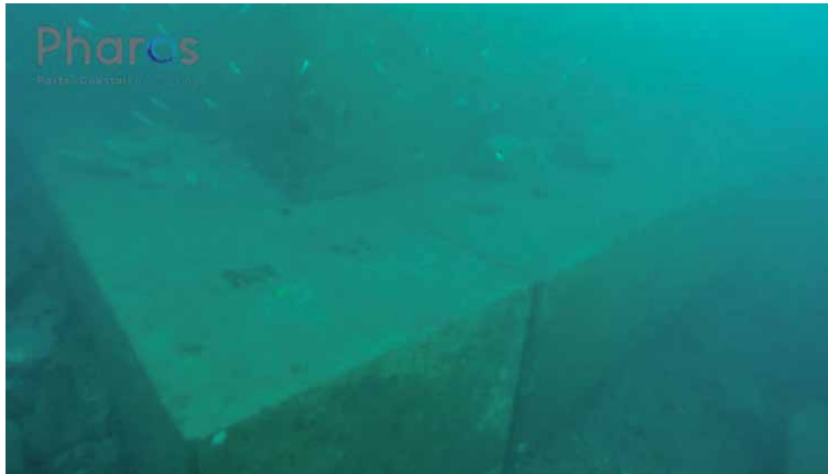
Figure 13. Detail of the foundation of the ramp.
