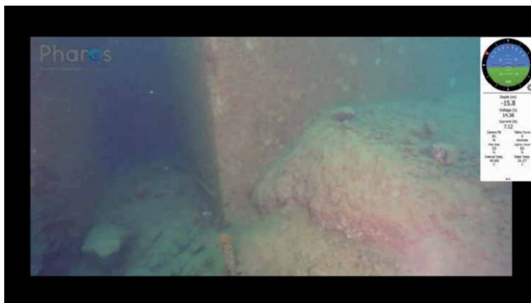
Figure 7. Detail of guard concrete executed in foundation.
