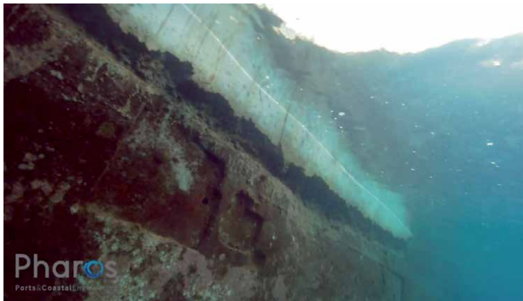
Figure 14. Ramp repair area.
