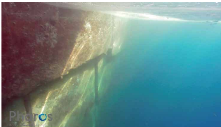
Figure 15. Vertical face of the ramp.
