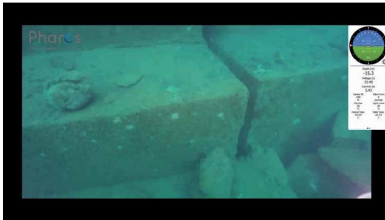
Figure 5. Quay blocks joint detail. Foundation footing.
