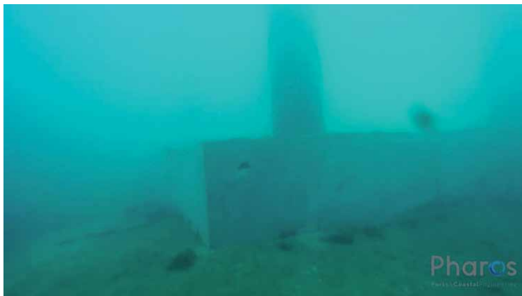
Figure 24. Duke of Alba's reinforced concrete foundation slab (Port of Naos).
