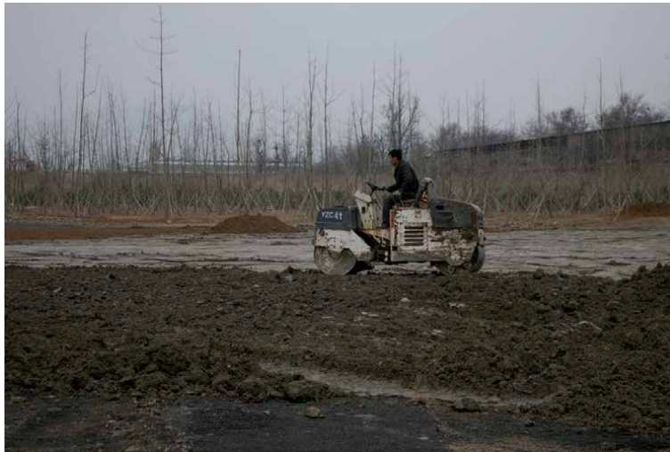
Figure 6. Use a tractor for site preparation.
