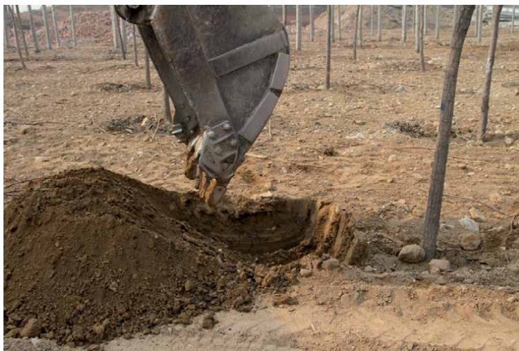
Figure 9. Use excavators to dig a hole for the afforestation.
